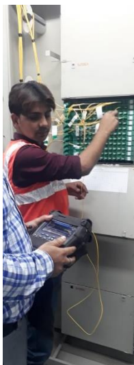
Delhi Central East OTDR Checking
