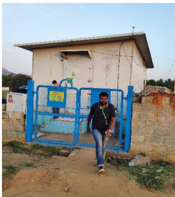
Equipment Location, Peenya
